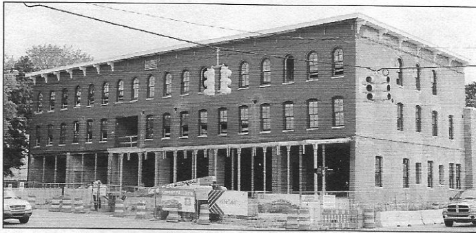
The Thompson Block renovation in progress.
