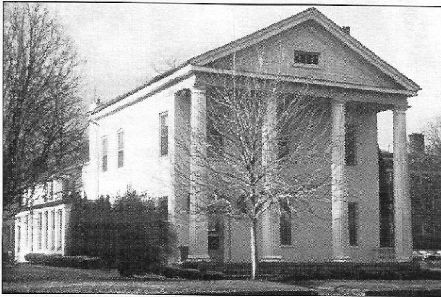
Ballard-Breakey House, 125 North Huron Street
