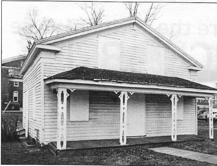
Towner House 1999 prior to exterior renovations.
