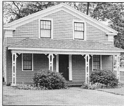
Towner House, 303 North Huron Street
