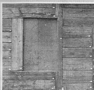
Left & above: Posted piece-sur-piece details
