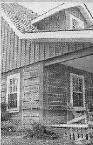
Posted piece-sur-piece construction is still used in modern building technology
