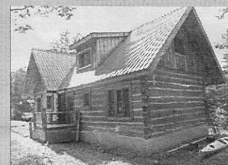
A modern keyed-log piece-sur-piece cottage in Quebec
