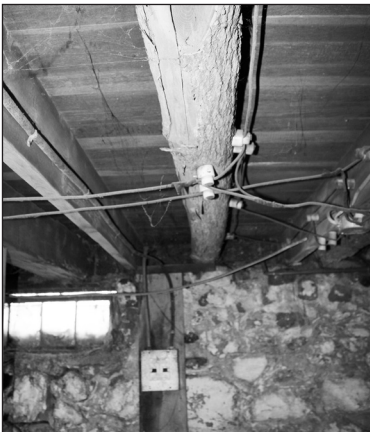
Interior shots of the Towner House as it stands today. Left photos shows the original timbers that still exist, knob and tube wiring and the Michigan basement foundation. Center and right photos show two of the first floor rooms that are in need of repair.
