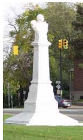
The joints were then tuck-pointed using a mixture of white silica sand, white Portland cement, and white lime. Instead of water in that mix, the liquid Don used was an acrylic mortar admix which increased bond strength and improved performance.
